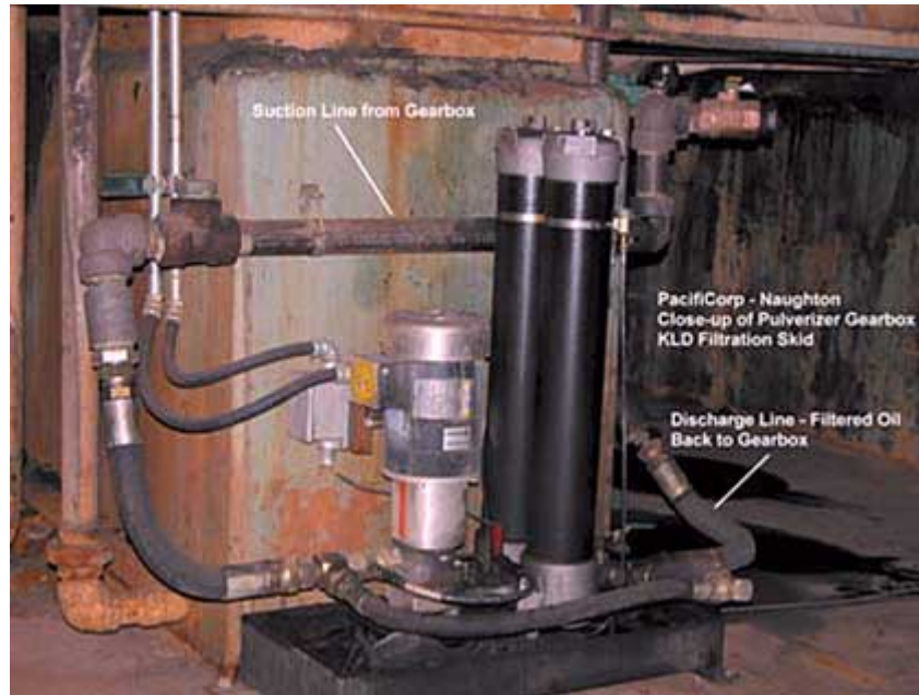
Figure 2. Kedney Loop Filtration System
